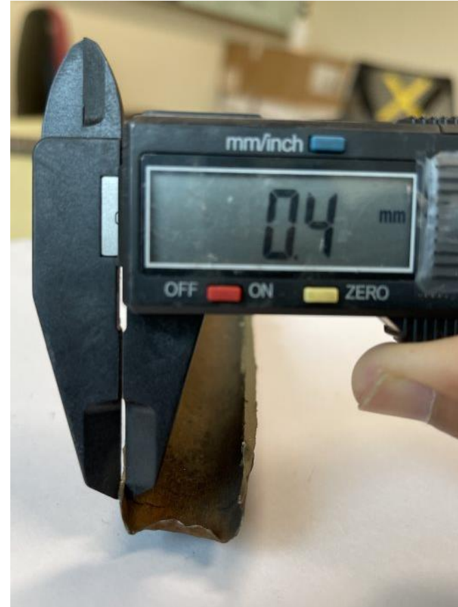
6. Thickness adjacent to sheared face
